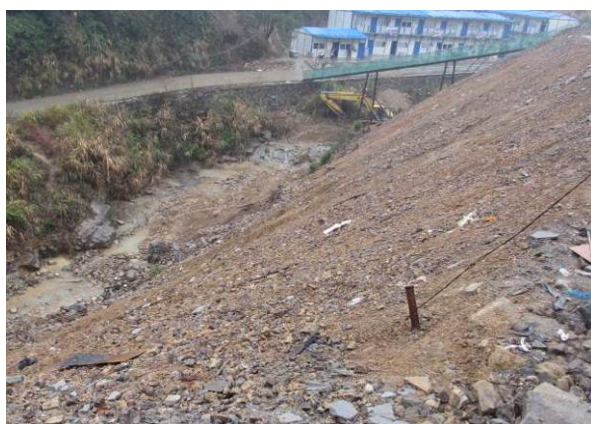
K6+200 处新填筑施工便道边坡
